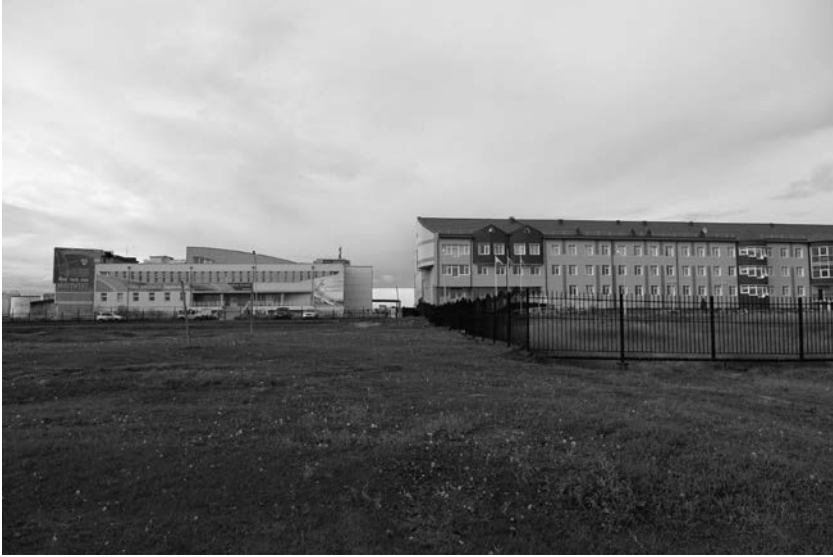
Figure 41a Institute of Physical Education and adjoining Sports School in Churapcha's regional center. Notice the ground already becoming uneven from thermokarst development (thawing permafrost). Photo credit: A. N. Fedorov.
