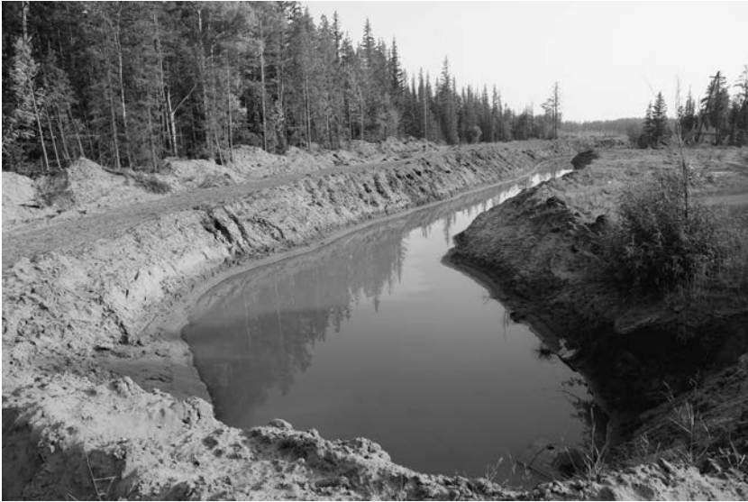
Figure 20 One of the many canals made in 2012–13 to drain flooded hay fields, with some so deep that livestock who accidentally fell into them drowned. Photo by author.
