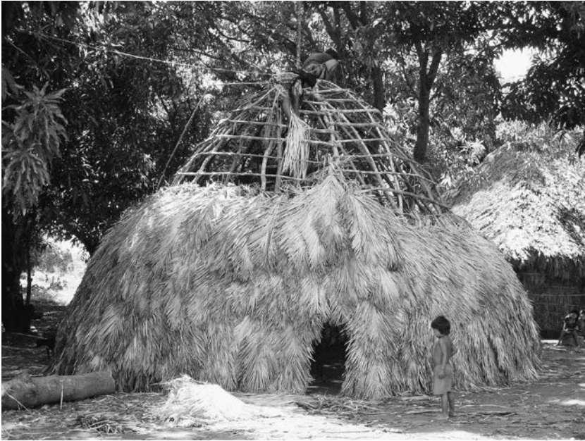
Figure 7 Photo of the author's house under construction on the east side of the Pimentel Barbosa community, 2004.
